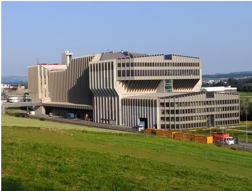
Fig. 6: Photo of the plant Renergia AG (Photo: Renergia)
